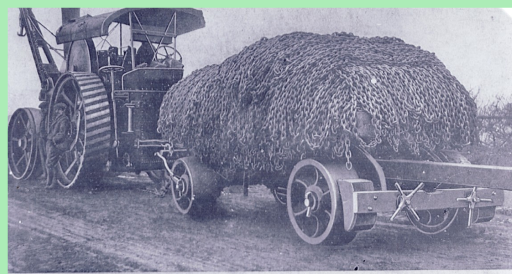
From MINE CHAIN, 11 inch diameter, length 200 yards, with 21 links, 10 lb. 3 oz. The chain was made by the Tinsley family in the Black Country. Makers - ELIZA TINSLEY & CO., OLD WELLS, SO.
