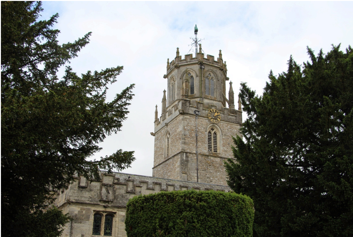
The parish church of St Andrew, Colyton.
