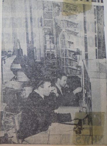
Above ground . . . G.P.O. technicians test circuits at a switchboard inside the new building. The workers are Alan Westwood and Bernard Frankham.
