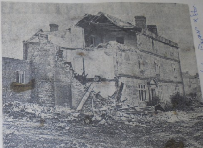
Gospel End House — partly demolished by mistake.
