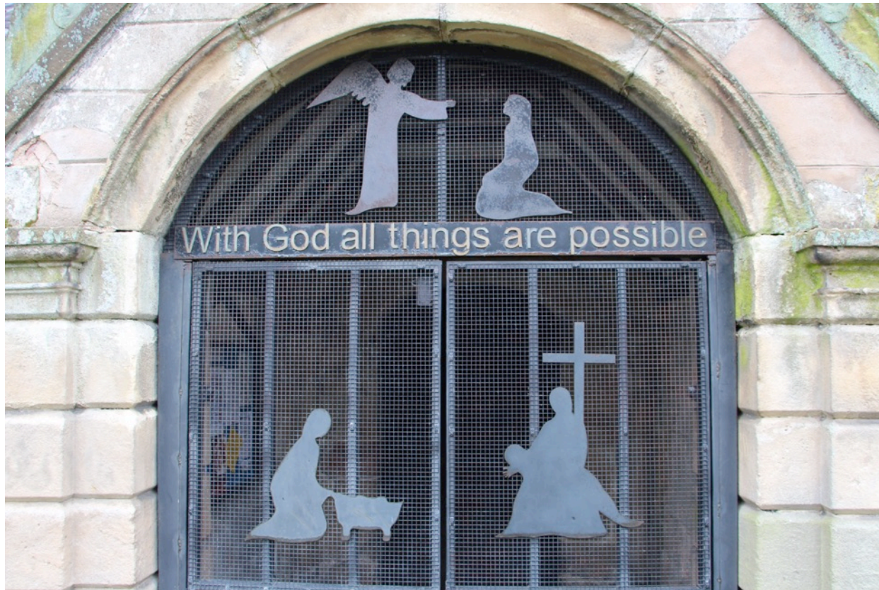
The outer doors to the porch at Shawbury – with cut steel figures.
