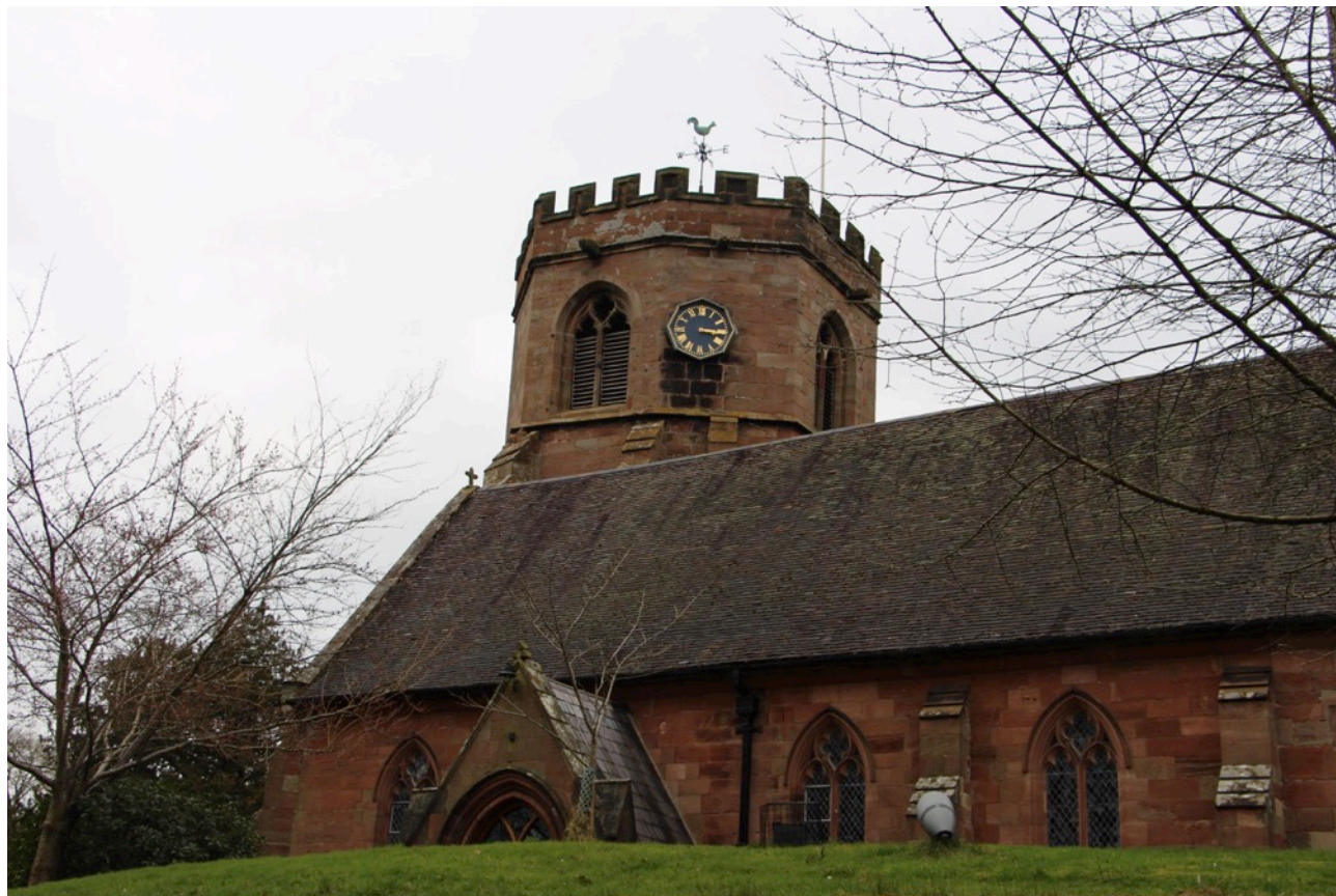
Hodnet – the octagonal tower.
