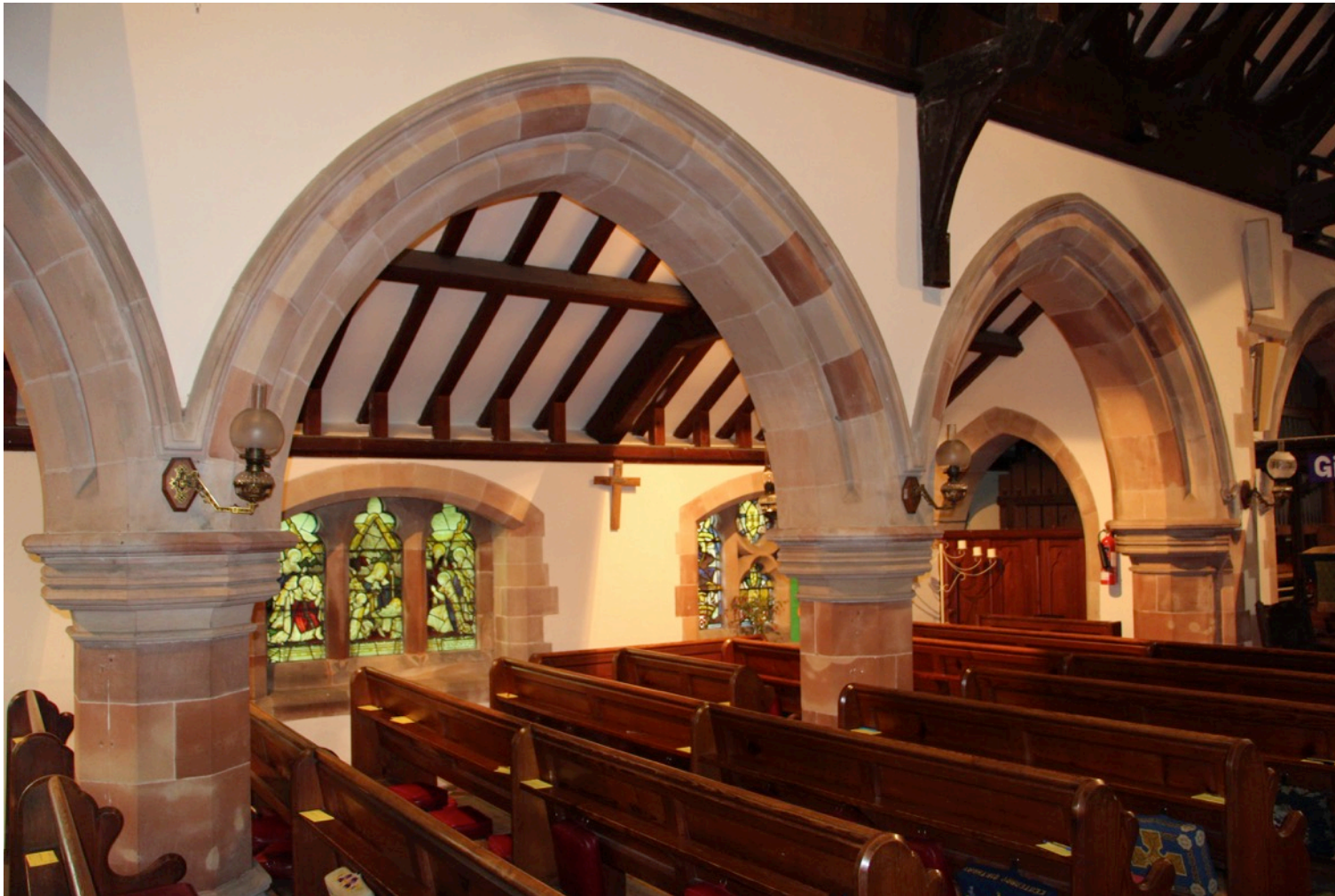
The nave and arches at St Michael, Ford.
