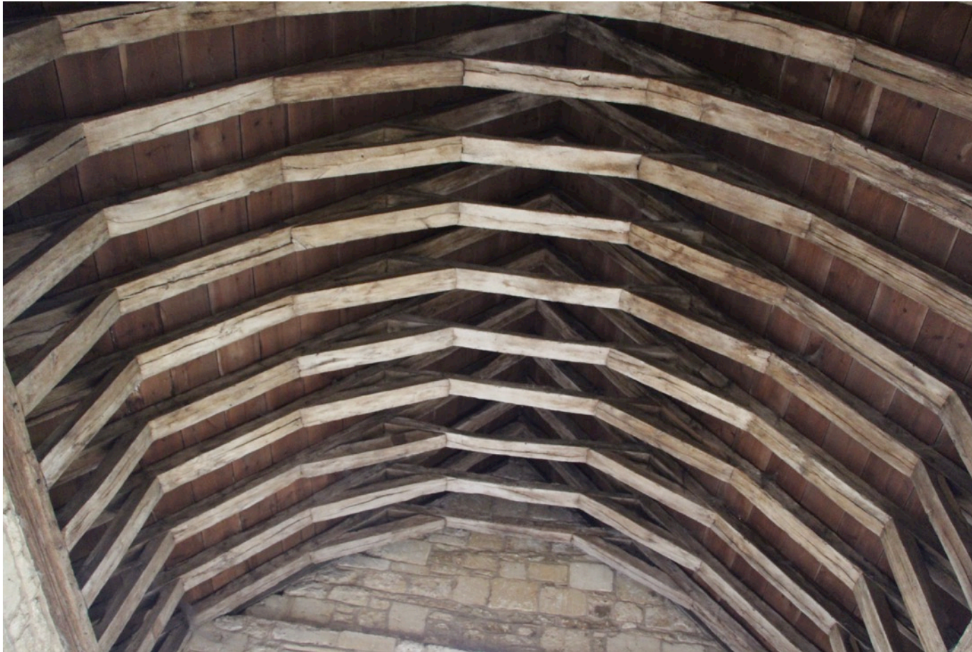
Roof timbers in the chancel at St Nicholas, Teddington, reminiscent of the construction of an inverted boat.
