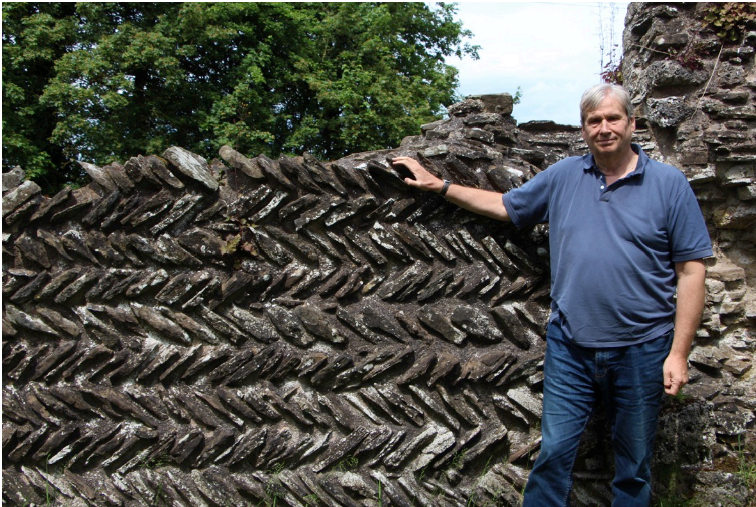
The astonishing herringbone pattern of the stonework at Edvin Loach Old Church. The herringbone-pattern stonework on the north and south walls is a feature of early Norman churches in this part of England.
