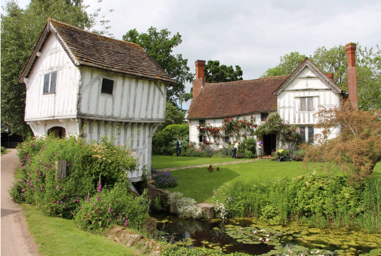
The unique timber framed Gatehouse and medieval Manor House at Brockhampton Estate.
