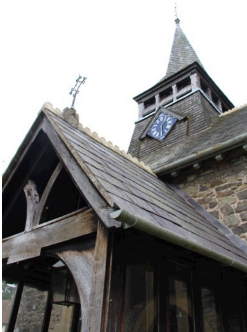
The wooden porch; and tower which contains a clock and three bells.
