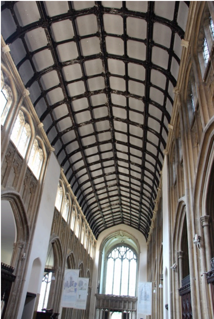
The roof at St Lawrence, Evesham.
